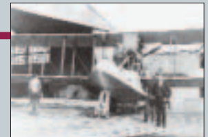
1920 — The first Coast Guard Air Station, operating with six Curtiss HS-2L flying boats borrowed from the Navy, was opened at Morehead City, N.C. The air station was closed after 15 months due to lack of funds.
